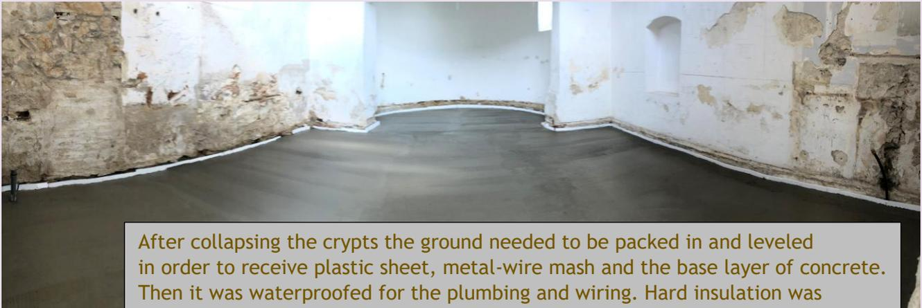
After collapsing the crypts the ground needed to be packed in and leveled in order to receive plastic sheet, metal-wire mash and the base layer of concrete. Then it was waterproofed for the plumbing and wiring. Hard insulation was installed with plastic sheet and another metal-wire mash for the underfloor heating pipes. The final step was C30 concrete, which is our final flooring as well. I cannot wait to see the diamond-grinded and polished floor...
