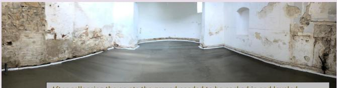
After collapsing the crypts the ground needed to be packed in and leveled in order to receive plastic sheet, metal-wire mash and the base layer of concrete. Then it was waterproofed for the plumbing and wiring. Hard insulation was installed with plastic sheet and another metal-wire mash for the underfloor heating pipes. The final step was C30 concrete, which is our final flooring as well. I cannot wait to see the diamond-grinded and polished floor...
